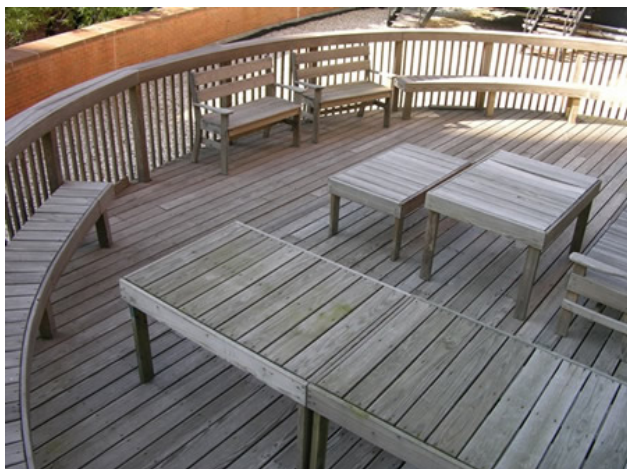
Hammer Building 2nd Floor Deck
